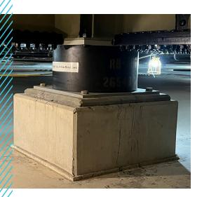
"These base isolators are kind of like massive hockey pucks with layers of steel through them. The building is isolated from the ground and can move 18 inches in each direction, which is pretty phenomenal," said Craig Stockbridge, principal, GBD Architects.
